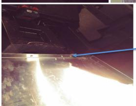
With the vertical slot of the pan bracket and the horizontal slot of the pan lined up place a 5/8" 1/4 #20 Phillips bolt with a washer through and attach supplied lock nuts.
